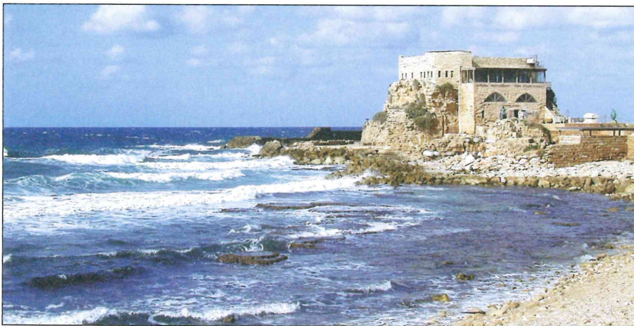
Herod's harbor in Caesarea was possibly the first port built in the open sea without the protection of bays and peninsulas. Two enormous, parallel breakwaters were built out from the coast into the sea.
